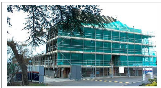
Refurbishment of the Old Building in progress
