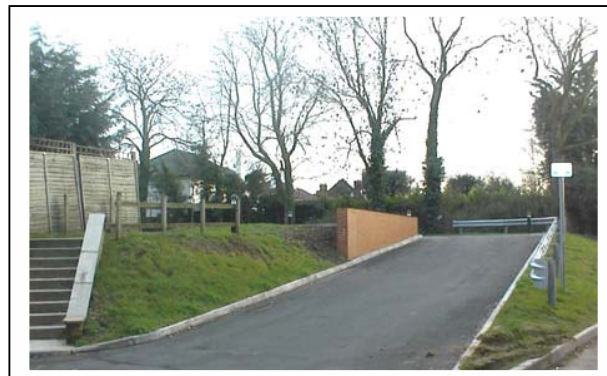
Ramp to new park on old tennis court Ramp to the new car park on old tennis court
