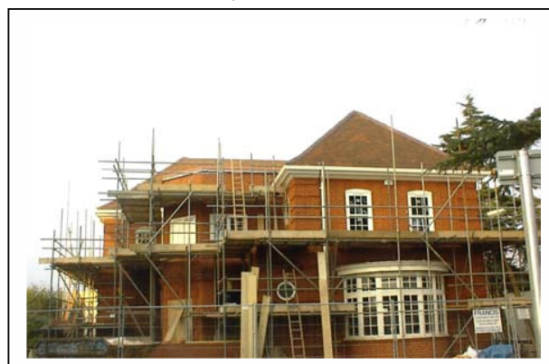
School House being renovated
